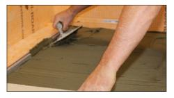
6 Apply a bed of tile adhesive to the surface of the dry screed, ensuring the front edge of the drainage channel has adhesive underneath it.
