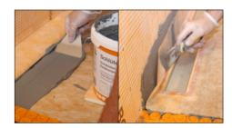
Adhere the Schlüter®-KERDI collar, using the sealing adhesive Schlüter®-KERDI-COLL-L (see Product Data Sheet 8.4), to the adjoining waterproofing assembly with a 3 x 3 mm or 4 x 4 mm notched trowel and comb provided. Completely embed the Schlüter®-KERDI collar in this assembly, observing the curing times of all materials.
