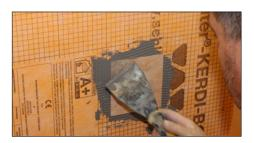
12 If Schlüter®-KERDI-BOARD is used on the wall, use Schlüter®-KERDI-COLL-L with a piece of Schlüter®-KERDI-KEBA sealing band to waterproof the penetrations.
