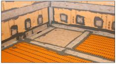
Use Schlüter®-KERDI-COLL-L to create tightly sealed wall connections with Schlüter®-KERDI-KEBA sealing band.
