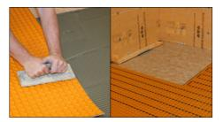
① If Schlüter®-DITRA 25 uncoupling membrane, or Schlüter®-DITRA-HEAT-E /-DUO underfloor heating is being used apply a bed of adhesive to the floor substrate and adhere the uncoupling membrane.
