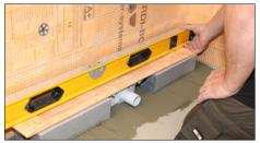
2 Using a spirit level adjust the drain until it is level along its length and across its width.
