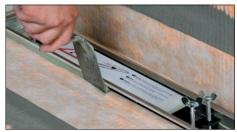
17 Use tile adhesive to fill beneath the frame on all sides and install the tile covering.
