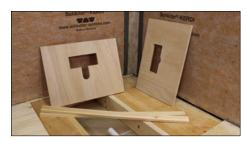
② Either construct and strengthen the subfloor in the section of the floor where the drain will be fitted or cut the pre-built 'G3 Installation Accessory 2021' to size. For guidance on constructing and strengthening the sub-floor see page 4. For guidance on using the pre-built 'G3 Installation Accessory 2021' see steps 10 to 13. We recommend using the pre-built 'G3 Installation Accessory 2021'.
