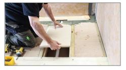
Place the remaining part of the sub-floor into position, screw fixing the shorter of the two pieces of plywood cut in step 16 to the battens. The longer piece should be placed on top of the lower piece and on top of the 'ledge' described in step C on page 4, or as part of the 'G3 Installation Accessory 2021'. The top piece should then be screwed to the bottom piece.
