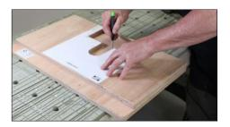
© Position the piece of sub-floor created in steps A & B over a further piece of 18mm exterior grade plywood, approximately 500mm long, lining up the ends of the plywood pieces that will be fitted nearest to the wall. Doing this will create a 'ledge' for the part of the sub-floor referred to in steps 16 & 21 to sit on and be secured to. Use the cut-out in the top piece of plywood to draw the shape onto the bottom piece of plywood.
