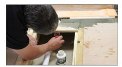
② Connect the drain outlet to the building drainage system ensuring an appropriate fall on the waste pipe. Check for leaks. Using a spirit level, check the drain is still level along its length and across its width, adjusting if necessary.
