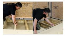
② Determine the position of the linear drain in the floor, taking into consideration the position of the floor joists and the size of the shower tray. The drain could be positioned either centrally or offset between the joists, but is usually positioned central to the shower tray width.
