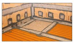
Use Schlüter®-KERDI-COLL-L to create tightly sealed wall connections with Schlüter®-KERDI-KEBA sealing band.
