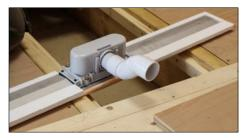
(E) Remove the drain and using solvent weld adhesive glue bends, as appropriate, to the outlet of the drain. One Floplast WS19 135° (45°) bend and one Floplast WS77 135° (45°) conversion bend usually works well.
