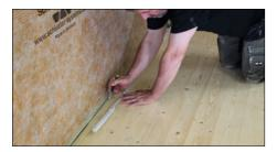
1 Identify and mark on the floor the position of the floor joists. The position of the screws or nails in the floor should provide an indication.
