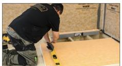
5 Check the width and length of the Schlüter preformed shower tray to be fitted and using a utility knife, cut to size.
