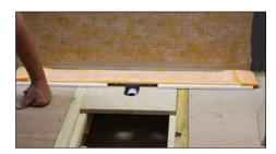
(b) Place the drain into position, with the drain body/sump sitting within the cut-out in the piece of sub-floor created as described on page 4 or within the cut-out in the 'G3 Installation Accessory 2021'.
