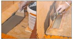
Adhere the Schlüter®-KERDI collar, using the sealing adhesive Schlüter®-KERDI-COLL-L (see Product Data Sheet 8.4), to the adjoining waterproofing assembly with a 3 x 3 mm or 4 x 4 mm notched trowel and the comb provided. Completely embed the KERDI collar in this assembly, observing the curing times of all materials.
