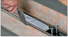
3) Use tile adhesive to fill beneath the frame on all sides and install the tile covering.
