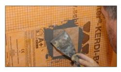
1 If Schlüter®-KERDI-BOARD is used on the wall, use Schlüter®-KERDI-COLL-L with a piece of Schlüter®-KERDI-KEBA sealing band to waterproof the penetrations.
