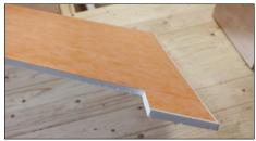
Using a utility knife and the pre-printed markings on the back, measure and cut out the sloped tray Schlüter®-KERDI-SHOWER KSLT13652000S to accommodate the drainage channel. If the drainage channel is fitted away from the wall ensure it still fits within the level end of the tray, and use either 12.5mm thick KERDI-BOARD, or the offcuts from the level end of the tray, to infill the gap between the wall and the tray.
