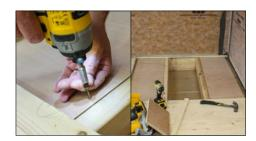
Screw fix the sub-floor to the battens, ensuring it is level. At this stage do not fix battens or the sub-floor to the area where the drain body/sump will be installed.
