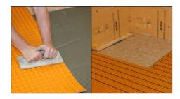
If Schlüter®-DITRA 25 uncoupling membrane, or Schlüter®-DITRA-HEAT-E /-DUO underfloor heating is being used, apply a bed of adhesive to the floor and adhere the membrane. As per Product Data Sheet 6.1, a 3 x 3 mm or 4 x 4 mm notched trowel should be used to install DITRA 25. As per Product Data Sheet 6.4, a 6 x 6 mm notched trowel should be used to install DITRA-HEAT-E/-DIJO.
