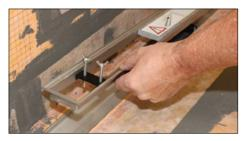
10 Insert the frame and spacer strip. If the 30mm high frame is being used (only suitable for use with a central outlet position) adjust the grate support around the trap to allow for cleaning.
