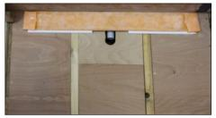
(6) Cut two further pieces of 18mm exterior grade plywood to fit, one on top of the other, in the remaining part of the sub-floor. Check they fit and then remove.
