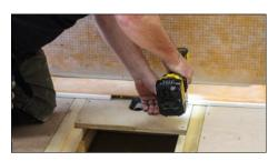
The strengthening the sub-floor as described on page 4 (and not using the pre-built 'G3 Installation Accessory 2021') screw fix it into the supporting battens described in step 8, ensuring it finishes flush with the top of the joists. Otherwise proceed directly to step 18.
