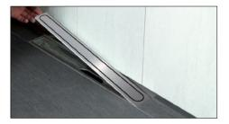
Remove the spacer strip and height-adjustment aid after curing. Insert the grate.
