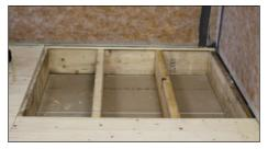
3 Carefully cut out the floor where marked, taking care to avoid any pipework or cables which may be in the floor void.
