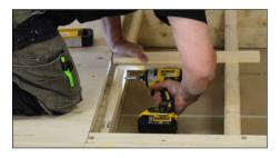
3 Using exterior grade 18mm plywood, construct the sub-floor where the shower tray and drain will be installed, fixing supporting battens to the floor joists at a depth so the sub-floor will sit flush with the top of the joists.
