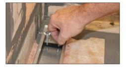
① Use the supplied height-adjustment aid to adjust the frame to the thickness of the tile covering.
