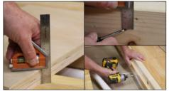
3 Fix supporting battens to the side of the joists in the section of the floor where the drain will be fitted. The top of the battens should be positioned 36mm from the top of the joists. Use screws sized to penetrate the joists by at least 10mm.
