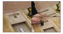
(E) Position the shorter piece of plywood over the longer piece secured to the battens in step 12, ensuring the routed-out section is face down and the cut-outs align. Glue the two pieces of plywood together (using a PVA-based D3 waterproof wood glue such as Gorilla Wood Glue) and then screw together. Use screws sized to penetrate the second piece of plywood by at least 10mm. Screws should be no further than 150-200mm apart across the whole of this piece of strengthened sub-floor.
