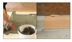
Using an appropriate notched tiling trowel, apply a bed of tile adhesive to the surface of the sub-floor where the shower tray will be installed. Carefully place the preformed shower tray on top of the adhesive bed, sliding the tray under the flange of the drainage channel. Ensure it is solidly bedded, adjusting the trowel size if necessary. Care should be taken to ensure the channel is not lifted.
