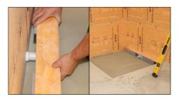
1 Having determined the position of the drain channel support and outlet, apply a thin layer of tile adhesive to the floor substrate where the channel support will sit. Embed the channel support in place ensuring good adhesion.
