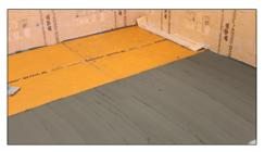
(5) If Schlüter®-DITRA 25 uncoupling membrane, or Schlüter®-DITRA-HEAT-E /-DUO underfloor heating is being used apply a bed of adhesive to the floor substrate and adhere Schlüter®-DITRA-25 uncoupling membrane, or Schlüter®-DITRA-HEAT/-DUO.
