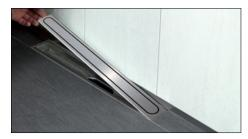
15 Remove the spacer strip and height-adjustment aid after curing. Then insert the grate.
