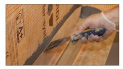
7 Adhere the Schlüter®-KERDI collar, using the sealing adhesive Schlüter®-KERDI-COLL-L (see Product Data Sheet 8.4), to the adjoining waterproofing assembly with a 3 x 3 mm or 4 x 4 mm notched trowel and the comb provided. Completely embed the Schlüter®-KERDI collar in this assembly, observing the curing times of all materials.
