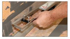
(2) Insert the frame with the spacer strip. If the 30mm high frame is being used (only suitable for use with a central outlet position) carefully adjust the grate support feet around the trap so the trap can be removed for cleaning.
