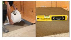
① Using screed create the slope (between 1 in 35 and 1 in 80) of the shower area, ensuring it is carefully installed up to and against the previously installed and levelled Schlüter®-KERDI-LINE-G3 drain.
