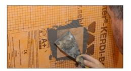
If Schlüter®-KERDI-BOARD is used on the wall, use Schlüter®-KERDI-COLL-L with a piece of Schlüter®-KERDI-KEBA sealing band to waterproof the penetrations.
