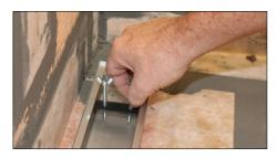
(3) Use the supplied height-adjustment aid to adjust the frame to the thickness of the tile covering.
