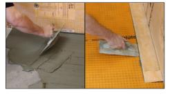
5 Once the screed is ready to bear weight, solidly embed Schlüter®-DITRA 25, or Schlüter®-DITRA-HEAT/-DUO underfloor heating, on the screed area with thin-bed tile adhesive (recommended notched trowel size 3 x 3 mm or 4 x 4 mm). The tile format for installation over Schlüter®-DITRA 25, or Schlüter®-DITRA-HEAT/-DUO underfloor heating, must be at least 5 x 5 cm (see Product Data Sheets 6.1 & 6.4).
