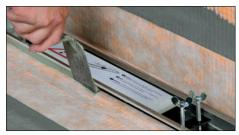
Use tile adhesive to fill beneath the frame on all sides and install the tile covering.
